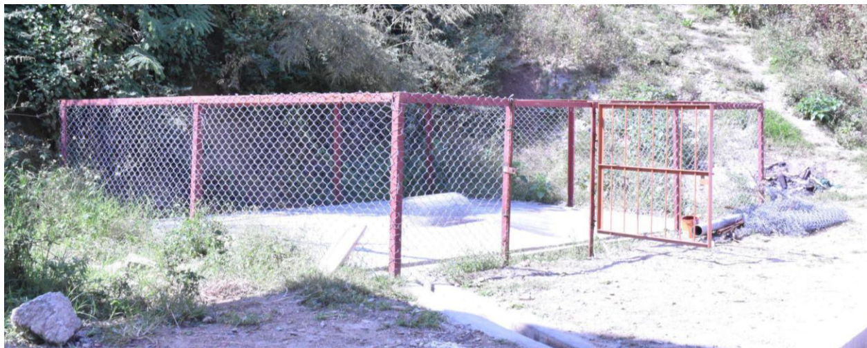
Figure 2: Deep burial pit in one of the PHC in Dagana.
