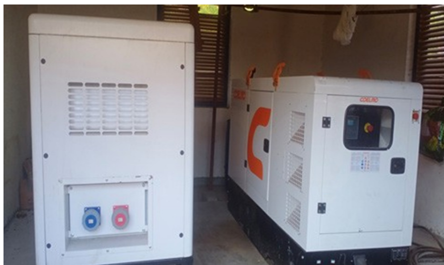
Generator used in EPI cold stores
